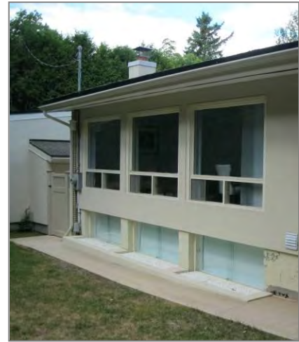
Figure 33: Horizontal sliding windows with sashless window units in the basement
