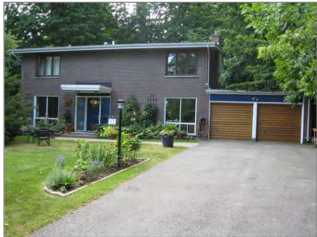
Figure 35: The front entrance at 12 Kindle Court features a wooden door, sidelight, spandrel panel, transom and a flat canopy.
